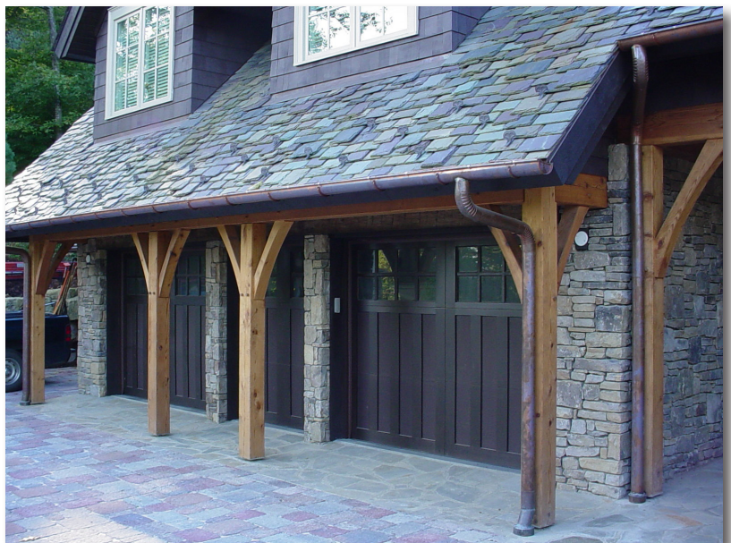
Cedar timber posts and braces
